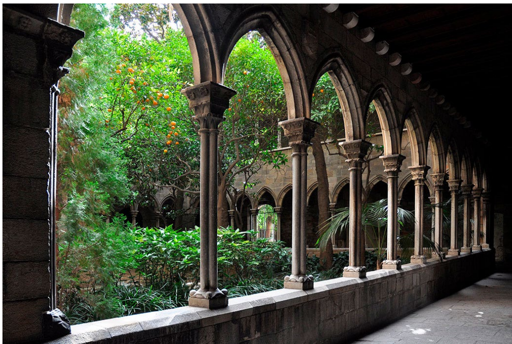
The Cloister. Today, more than two hundred people in need are provided with lunch and dinner every day, in addition to medical services and companionship.
